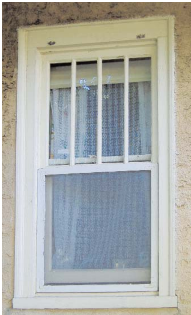
While the owner of this house spent extra money on this replacement window (left) for a custom muntin pattern to match the original (center), the stark white color, shallow muntin depth and lack of divided lites fail to convey the feel of the original. The trim around the replacement window was also capped with aluminum, another “no maintenance” effort that ruins the appearance of the window (notice the loss of the backband surrounding the trim). It will create a long-term problem when water trapped behind the aluminum rots the wood beneath. A level of thermal resistance comparable to that of a new window can be obtained by adding a storm window to the original (right).
