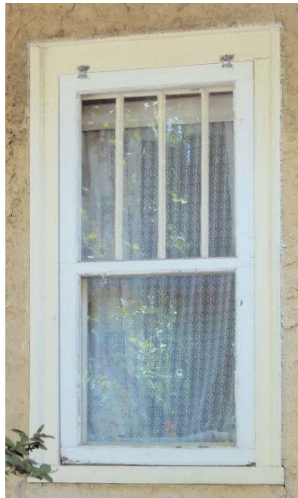
While the owner of this house spent extra money on this replacement window (left) for a custom muntin pattern to match the original (center), the stark white color, shallow muntin depth and lack of divided lites fail to convey the feel of the original. The trim around the replacement window was also capped with aluminum, another “no maintenance” effort that ruins the appearance of the window (notice the loss of the backband surrounding the trim). It will create a long-term problem when water trapped behind the aluminum rots the wood beneath. A level of thermal resistance comparable to that of a new window can be obtained by adding a storm window to the original (right).
