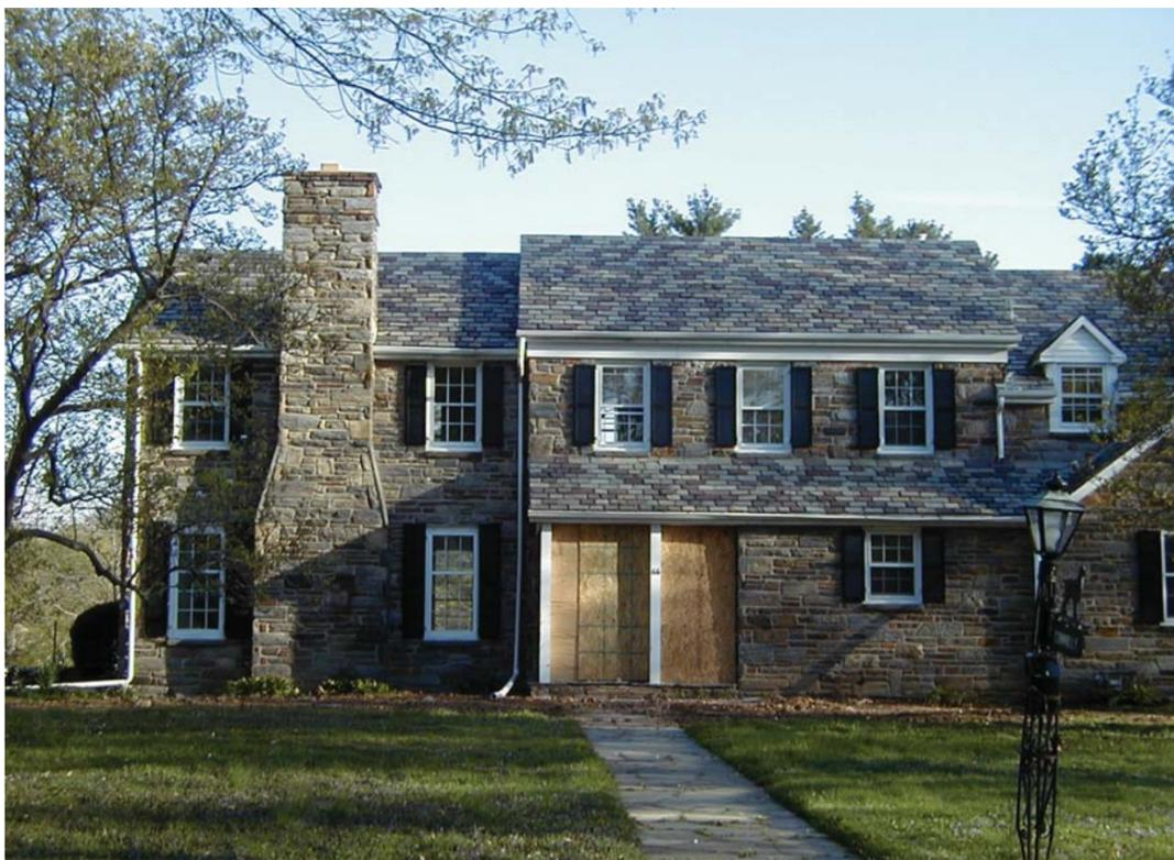
Asphalt shingles (top) are not capable of emulating the thickness, texture and variegated color of slate (above).
