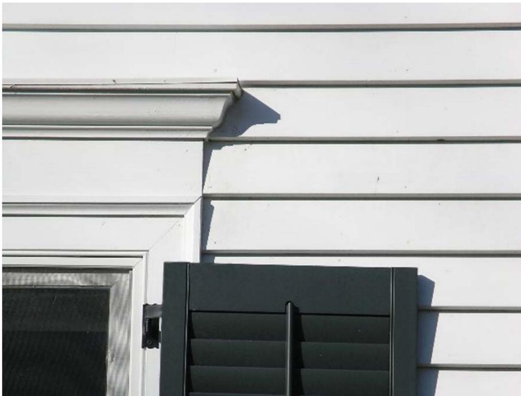
Faux wood graining, J-channels around windows and aligned and overlapping butt joints reveal this vinyl siding (top) to be a poor imitation of cedar siding (above). All photos courtesy of John Cluver, Voith & Mactavish Architects
